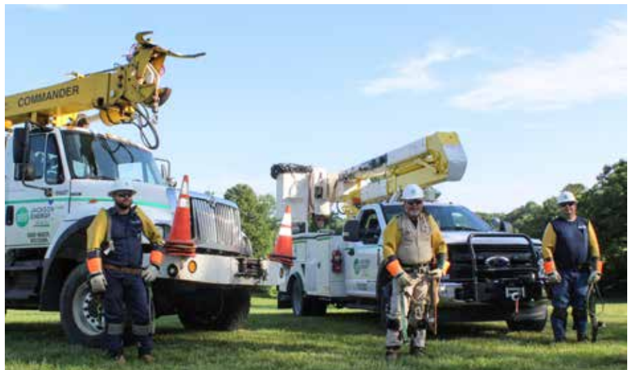
Jackson Energy's 1st Class Line Technician Brandon Keyton, Service Technician Mike Truett and Service Technician Kris Cunagin prepare to restore service after a thunderstorm ripped through Jackson County. Photo: Lisa Baker
