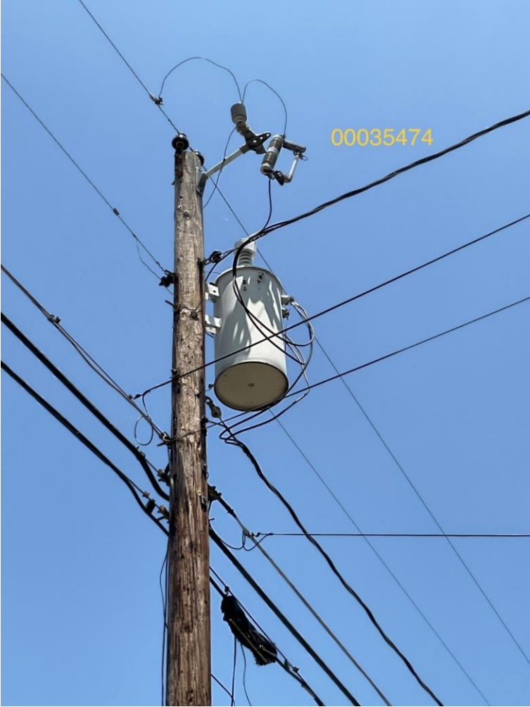
Figure 5.1: Communications attachments are too close to the lowest power on the pole (service/bottom of electric transformer)
