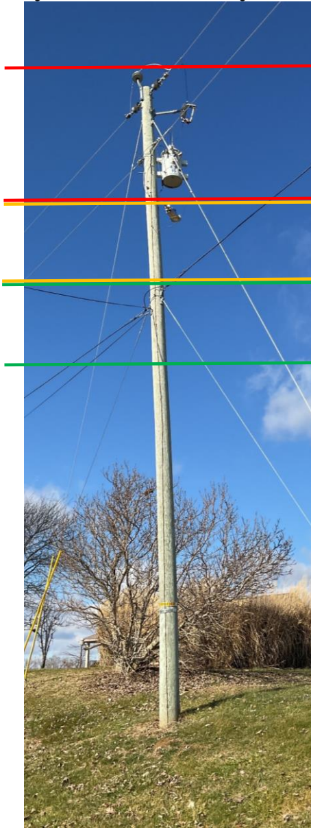
Figure 1 – Distribution Pole with working zones identified
